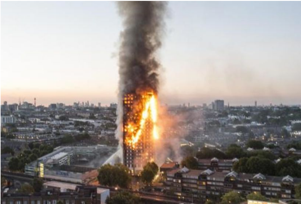
Grenfell Tower Fire Jun. 2017
